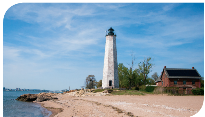
Lighthouse Point Park, the western terminus of the Shoreline Greenway Trail.
